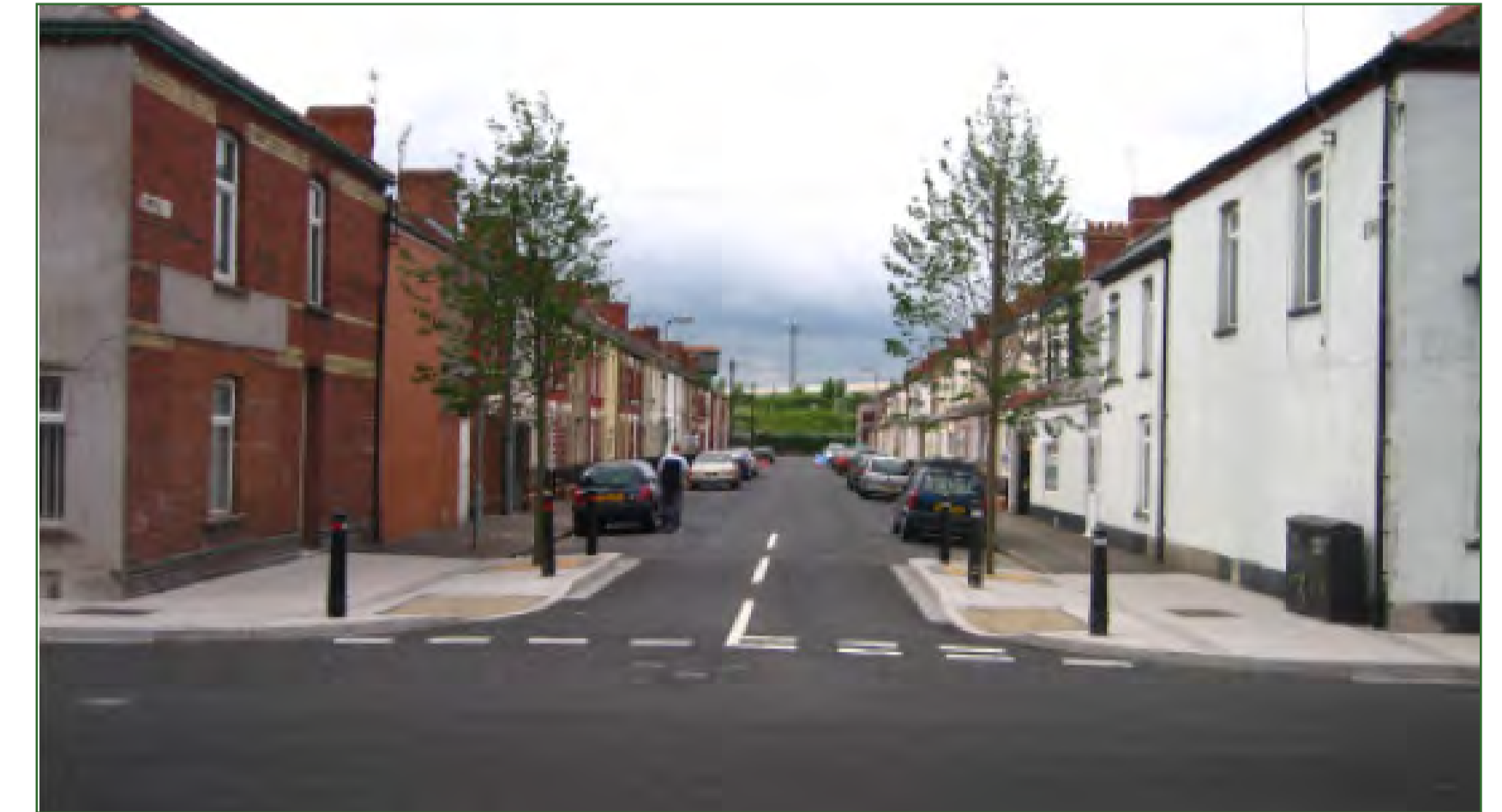
Reducing the turning space for cars at a corner to allow easier crossing.
