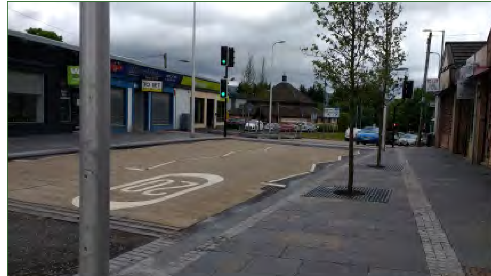
Limiting road space to slow down car movement and give more room to people and cyclists.
